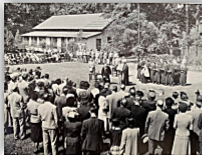
Groundbreaking for the Education Building, September 25, 1949. Note President of SC Synod, Karl Kinard (Porter Kinard’s father) in top picture on right.
